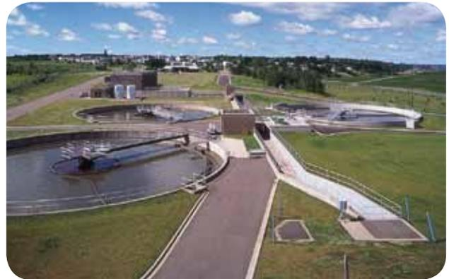
The actual WWTF was commissioned in 1994 with a capacity of 115,000 m<sup>3</sup> per day, or 25 million gallons per day. The plant was laid out to facilitate expansion to biological treatment in the future.
