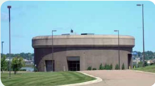
The Main Pumping Station located on the plant site at Outhouse Point (property having been granted initially to a Mr. Robert Outhouse) is the heart of the collector sewer system, a point of collection for all lines and continuous pumping to the Wastewater Treatment Facility (WWTF). The cylindrical structure extends 30 m below grade and 9 m above ground, much like a 10-storey building underground.
