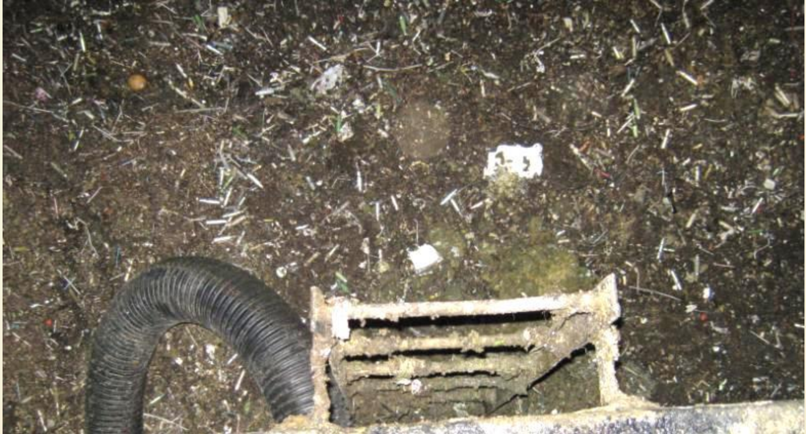
Cleaning of wet well.
