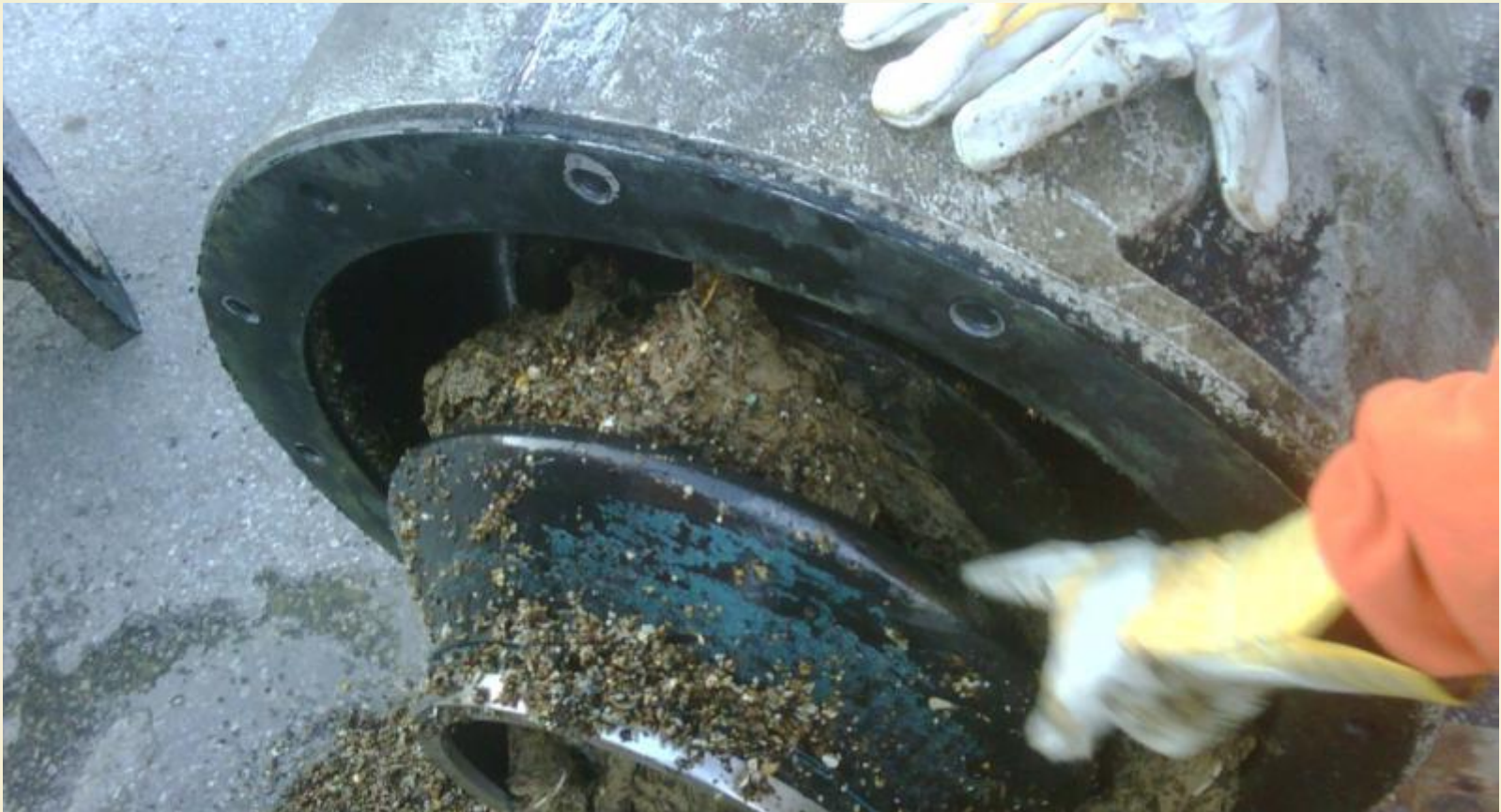
Cleaning out of pump.
