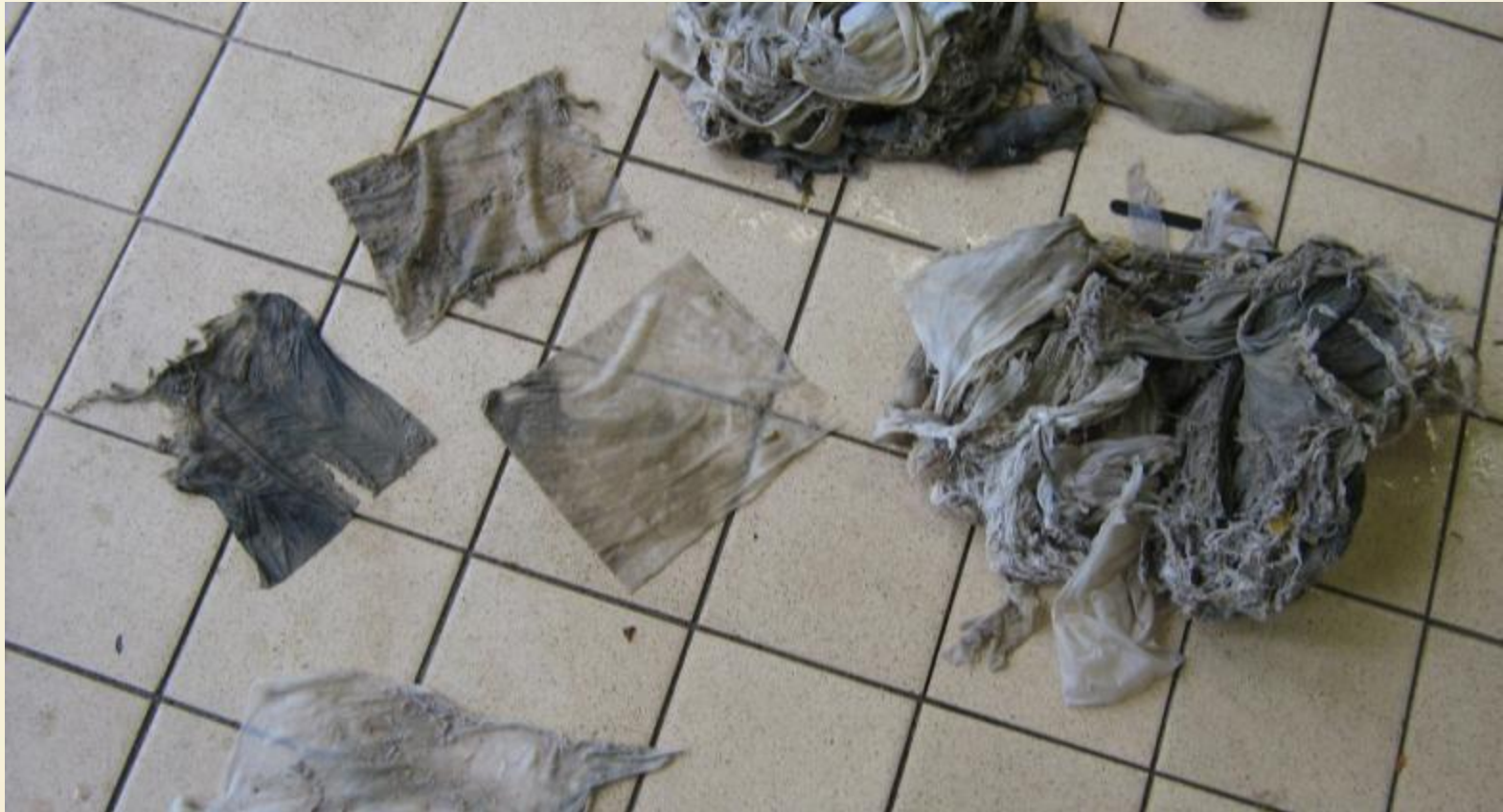
Investigation of plugged pump.
