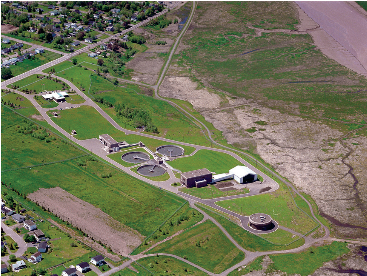
Aerial view of GMSC's Wastewater Treatment Facility in Riverview.
