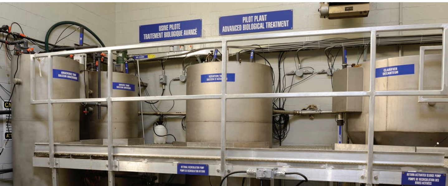
Biological nutrient removal GMSC Pilot Plant.
