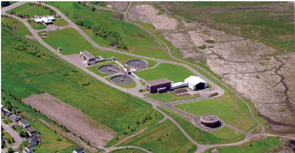
Aerial view of TransAqua’s Wastewater Treatment Facility in Riverview.
