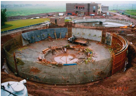
Clarifier under construction.
