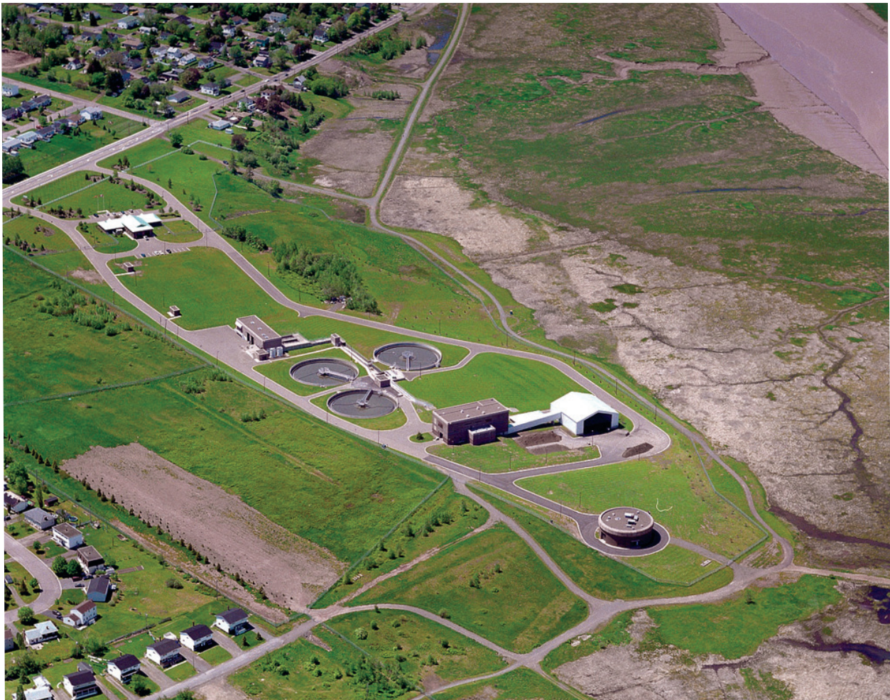
Aerial view of TransAqua's Wastewater Treatment Facility in Riverview.
